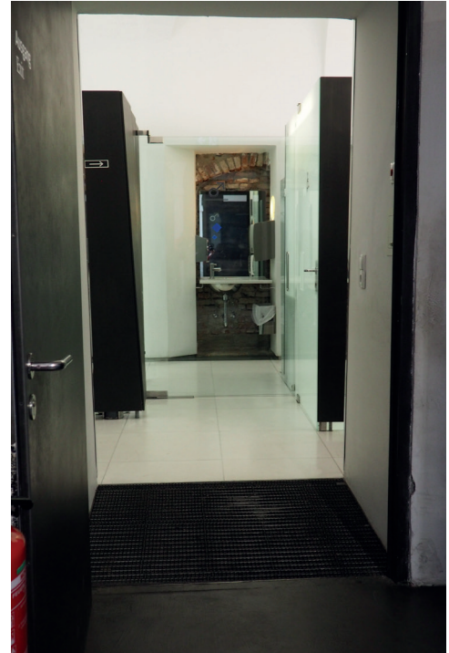
Access to the WCs, 6 % gradient
